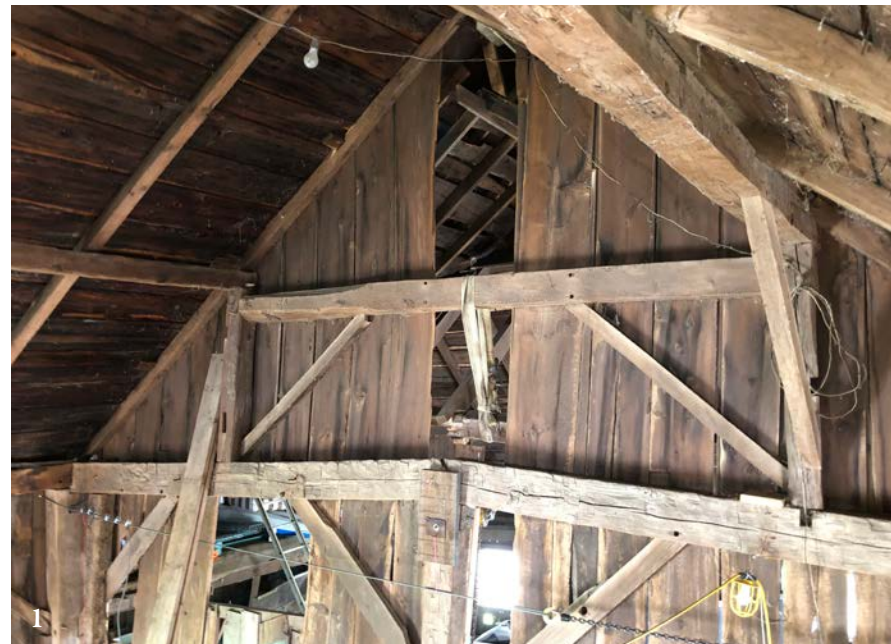
1 The west gable of the 1794 barn illustrates the condition of the barn as found. It was definitely in need of some help. The wider, lower braces were riven, the upper braces up-and-down sawn.
